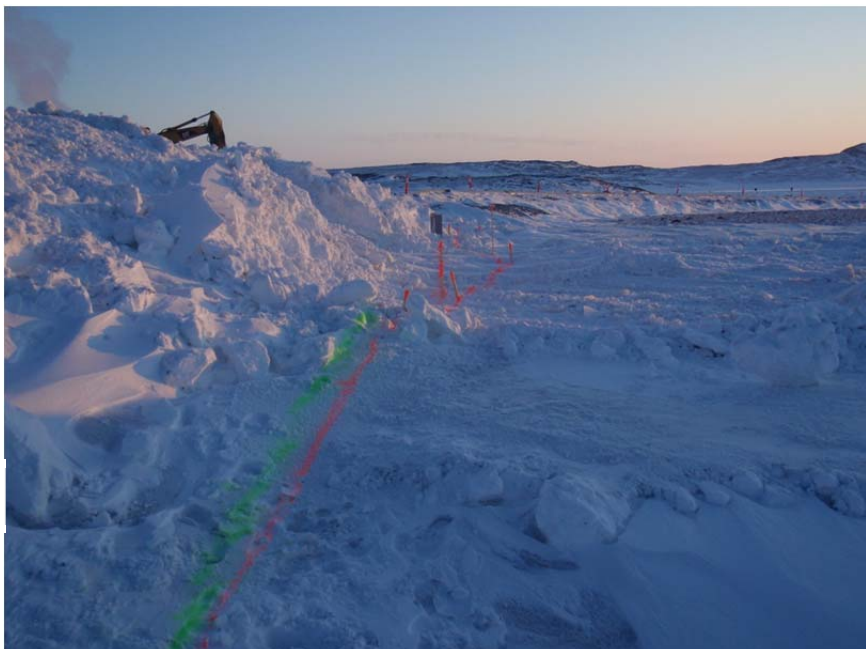
Photo 15: ~E view towards the Doris Camp Sump #1. Note that the green and orange spray-paint marks the as-built location of the cables which intersect the Sump #1 footprint.
