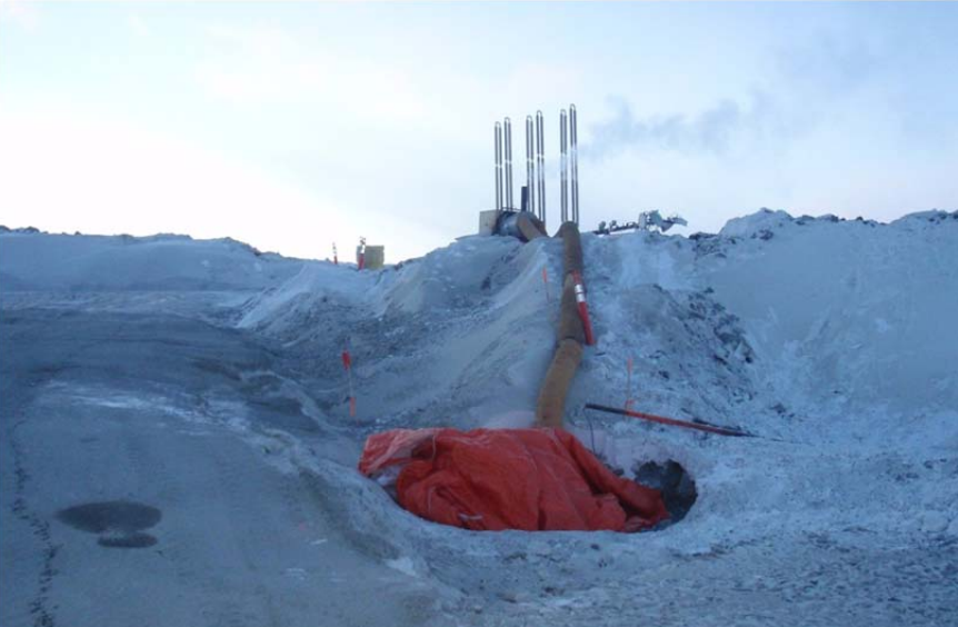
Photo 4: ~ NWW view of hording and frost fighter set up to warm thermistor string ND-HTS-060-28.8 for repair.
