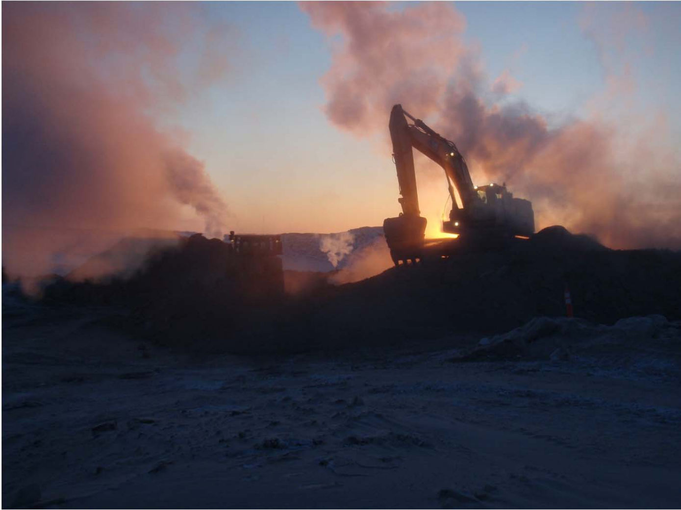
Photo 1: 345 excavator and D8 dozer working on breaking up unsaturated lumps of FCM at the stockpile on the FCP pad; ~W view
