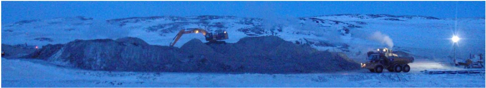
Photo 9: ~NE view towards the FCM stockpile on the FCP pad. Note the 345 excavator, 730 haul truck and loader working on breaking up the frozen stockpile.
