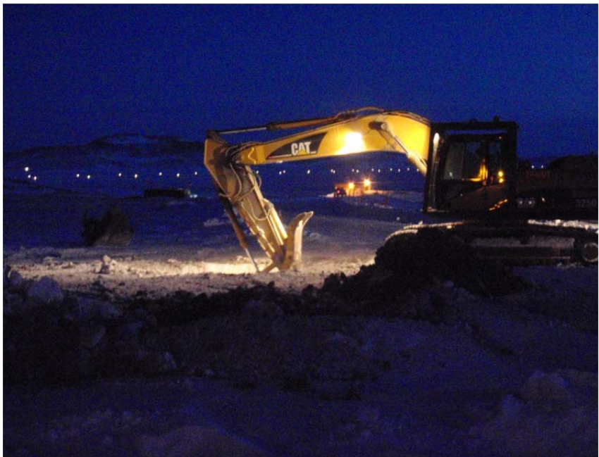
Photo 16: ~E view of the 325 excavator (with toothed bucket) working on excavating material from the drilled Sump #2 footprint.
